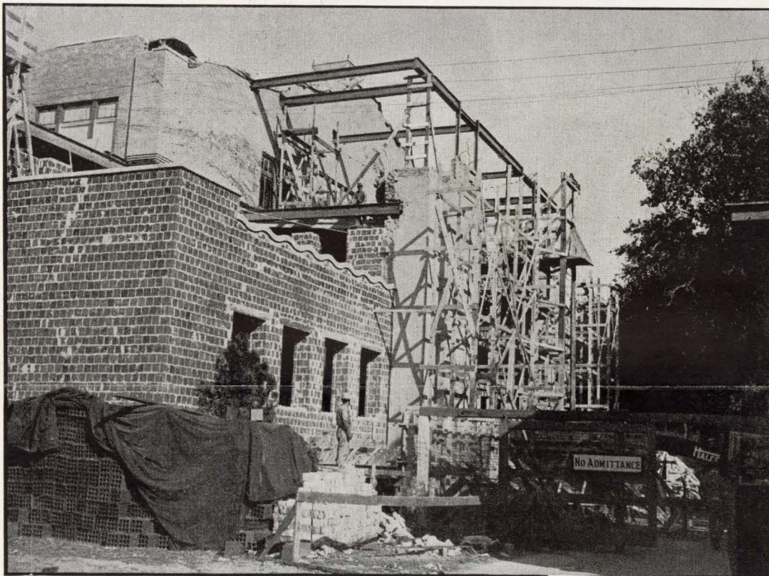
Construction of Texas Centennial Exposition Administration Building (upper left) nears completion.
