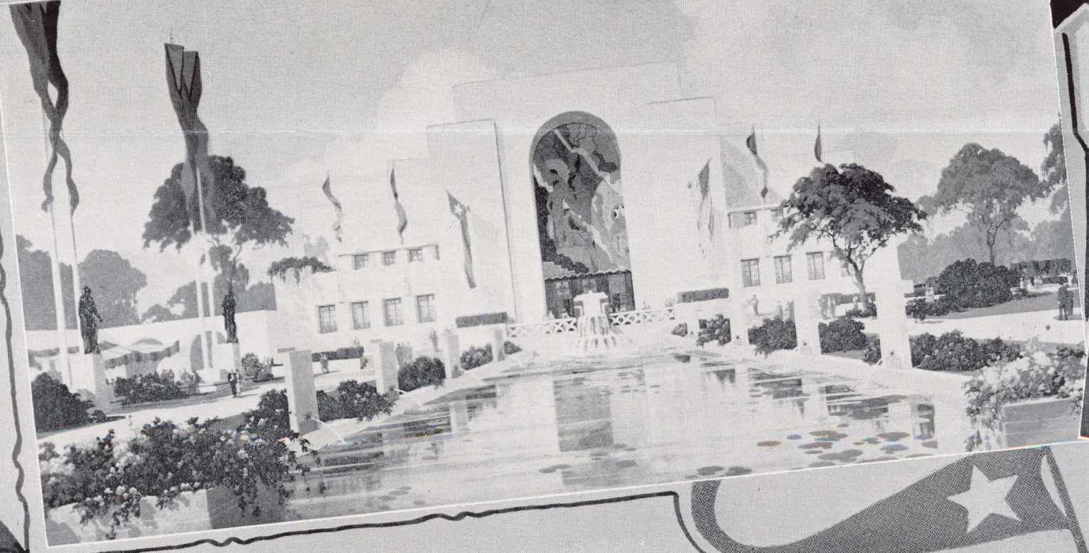
The influence of early Aztec period in Texas history, combined with the classic modern trend of today, will be seen in buildings of the 1925 Poultry and Agriculture Buildings; center, the $1,200,000 State of Texas Building; lower left, A
